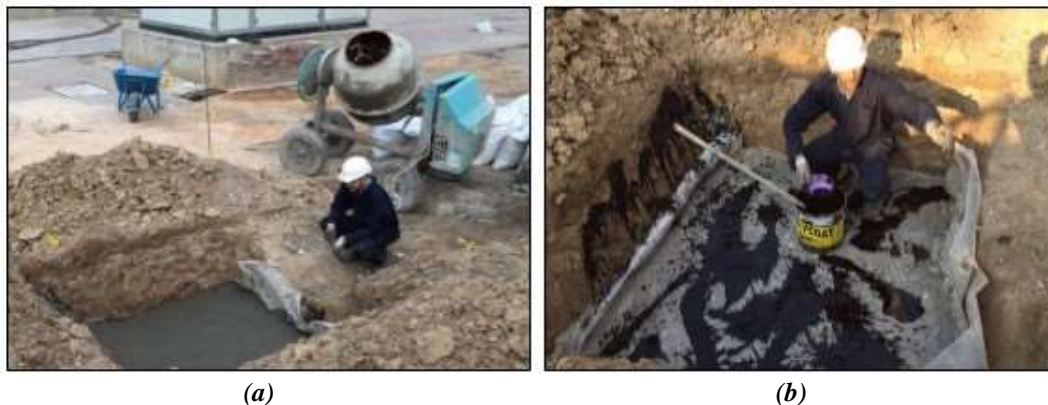
Figure 3: Field model preparation at the University of Technology and placement of the concrete mix slab.
